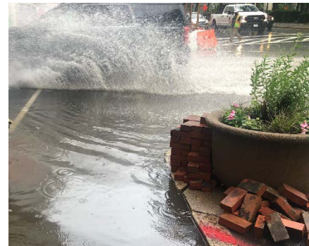
Figure 3 A flooded street and crosswalk. Source: Amanda Farber
